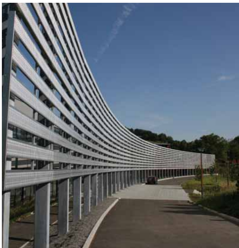
© Architecture-Studio - St-Étienne Métropole - Service communication
